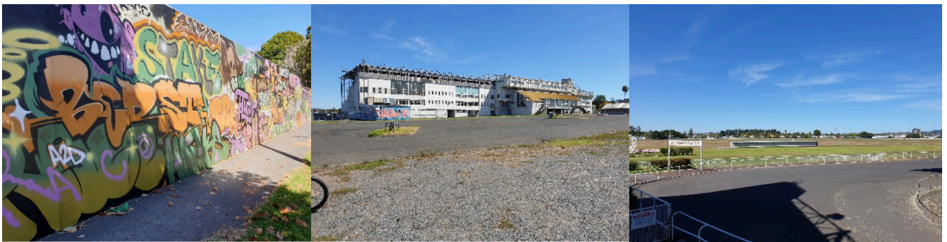
Figure 46: Avondale Racecourse showing dilapidated buildings, fields, and graffiti on fencing.
