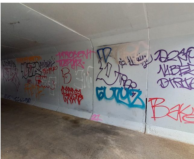
Figure 25: Alderson Road underpass and entrance.
