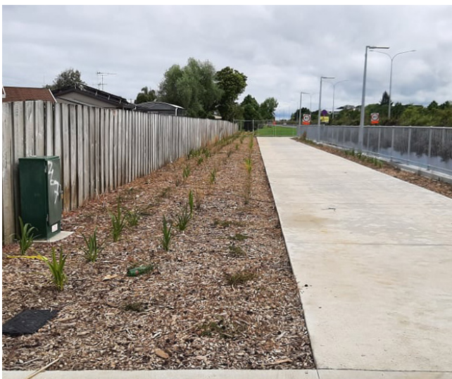
Figure 33: Underpass entrance footpath.
