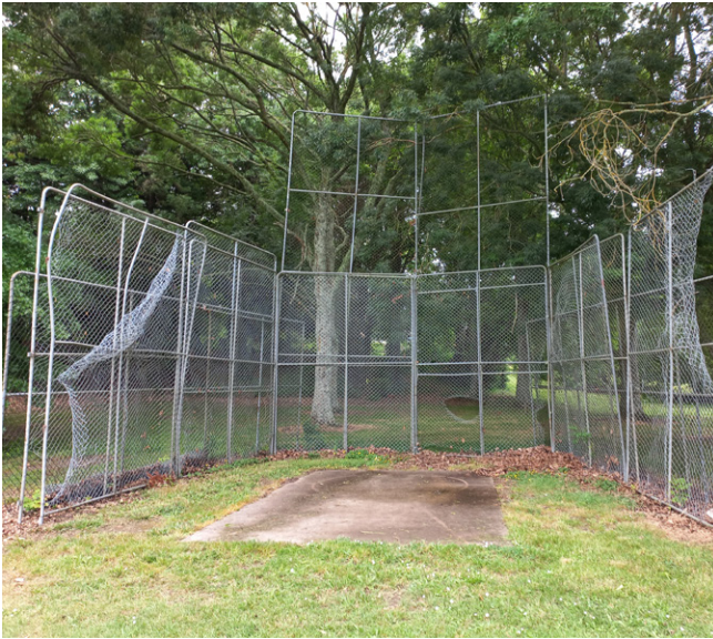
Figure 21: Old Porritt Stadium Throwing Cage. A tree has fallen on the cage during the cycle further damaging it.
