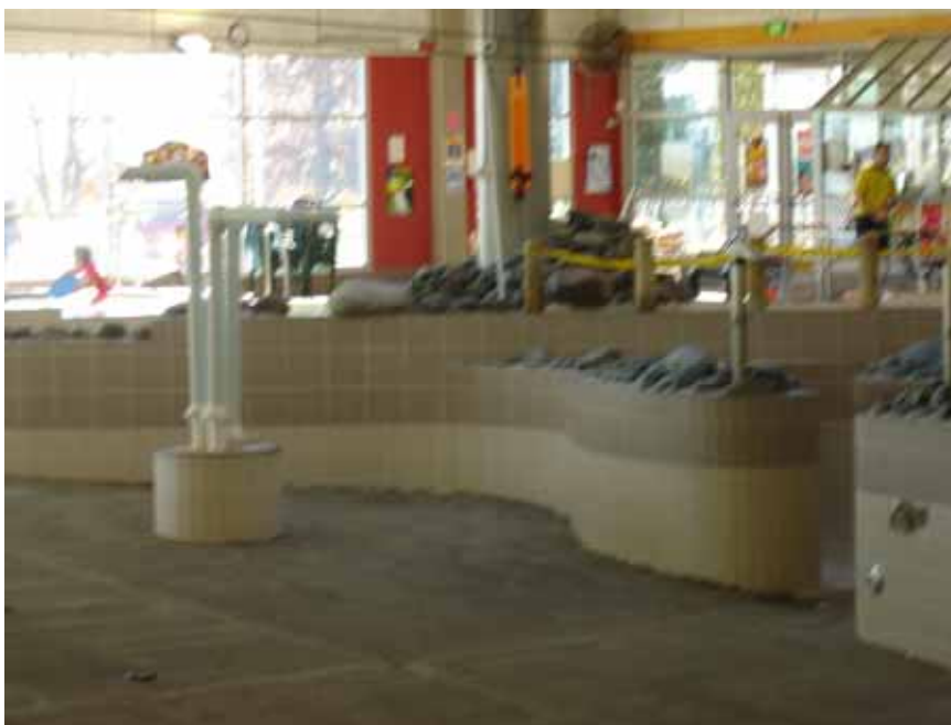
Richmond Pool under repair
