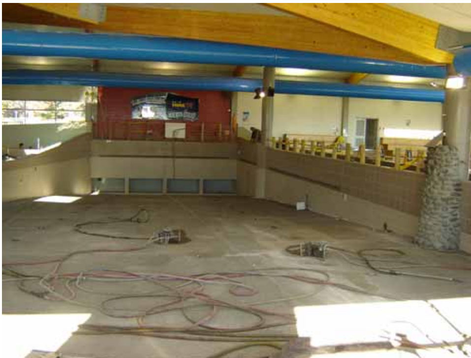
Richmond wave pool tile replacement
