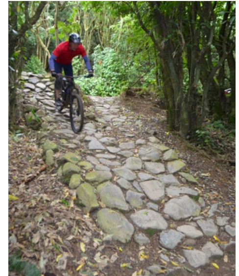
Rock armouring at the top of Starfish, Makara Peak, Wellington.
