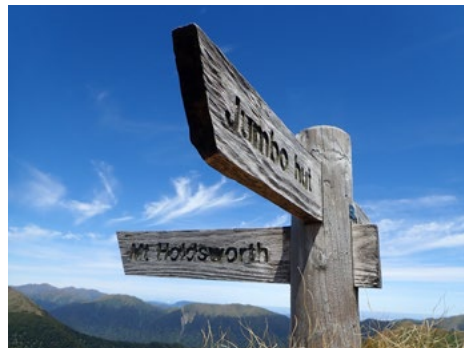
Wooden routed fingerboard signs that have lasted for over 30 years at 1400m elevation.
