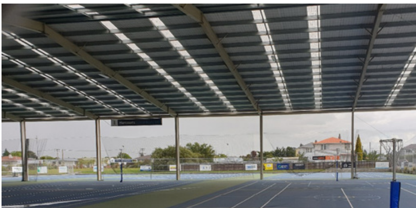
Masterton Netball Centre has transparent panels to improve natural light
