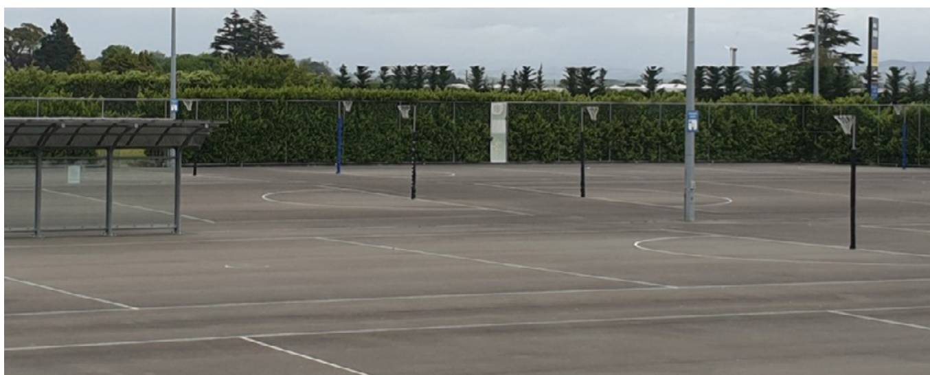
HAWKE'S BAY NETBALL CENTRE, MITRE 10 PARK WITH CROSS FALLS OF 1:90 AND LONGITUDINAL FALL APPROXIMATELY 1:500.
