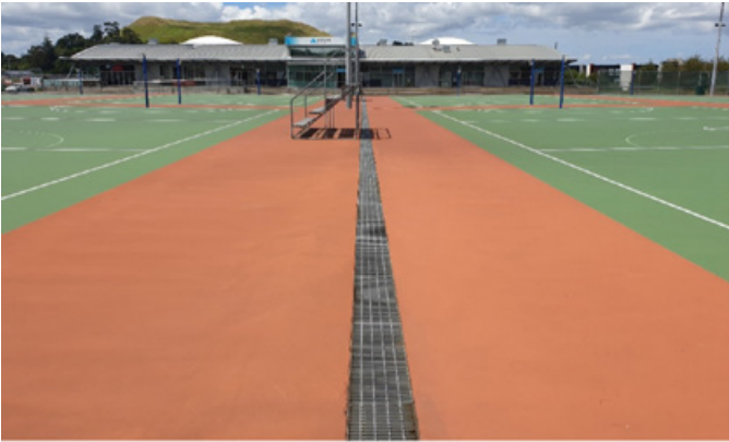
Dish-drains and good cross-falls help deliver dry courts.
