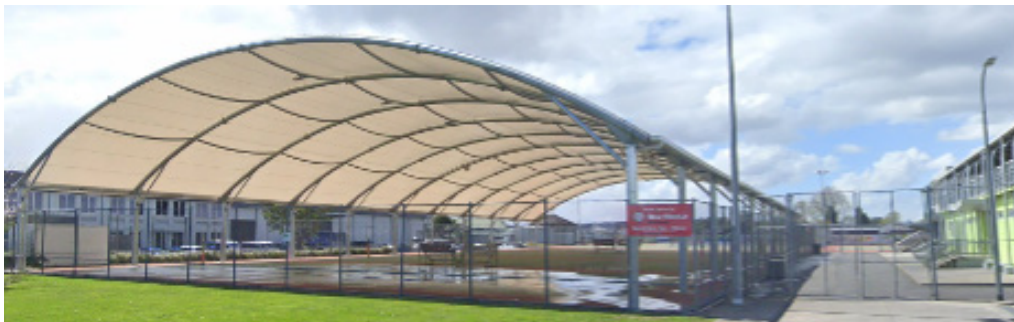
Manurewa Netball Centre has 5.5 metre pole height and 11 metre centre.
