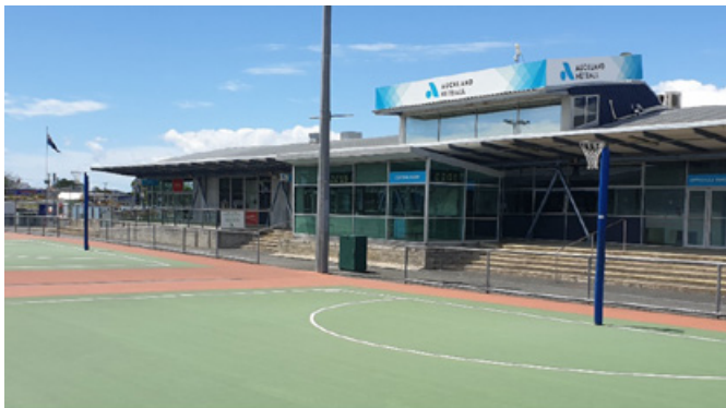
Auckland Netball Centre initially designed a lower and upper control room, but only use the lower control room on game day as it is more connected and accessible. The all glass design is challenging to keep warm in winter and cool in summer.
