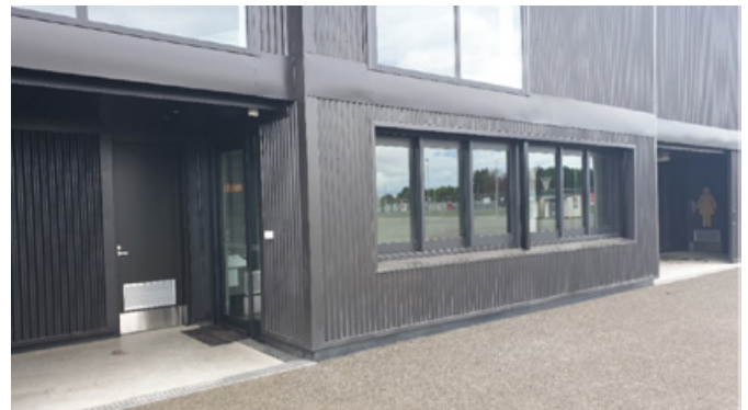
Marlborough Netball Centre has a large ground floor control room as part of the Lansdowne Sports Hub with good windows and participation interface.
