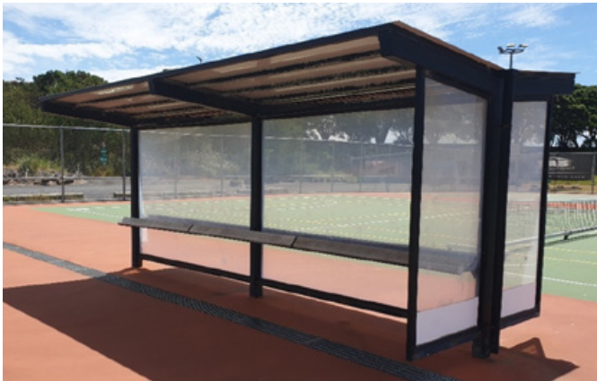
Auckland Netball Centre shelters
