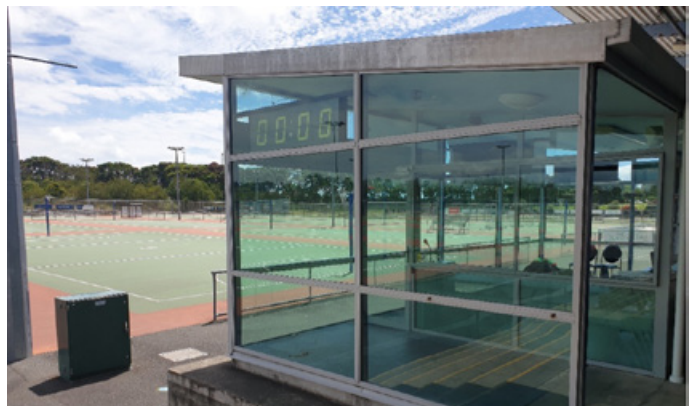
The control room is located on the ground floor connected to play. The all-glass construction can be difficult to regulate the temperature.
