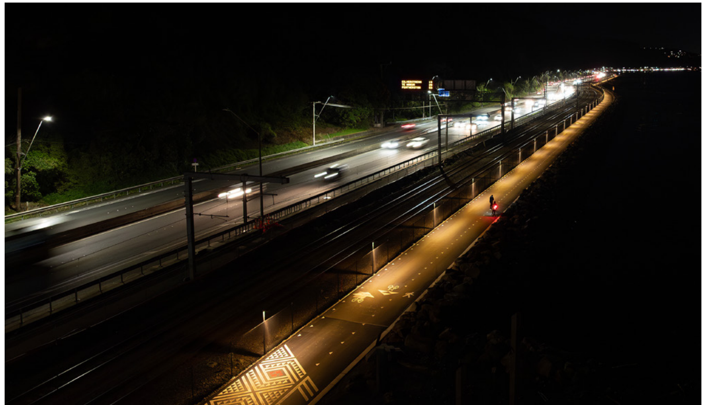
Te Ara Tupua at night, Te Whanganui-a-Tara Wellington to Te Awa Kairangi ki Tai Lower Hutt.
