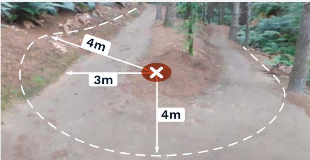
◀ Diagram 7: Correctly measuring a turning radius to mark out accessibility enhancements.
