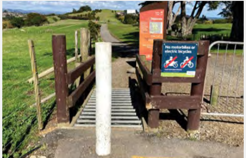
▲ Photo example: a bollard with narrow spacing either side positioned at the start of a narrow cattle stop with fencing either side.
