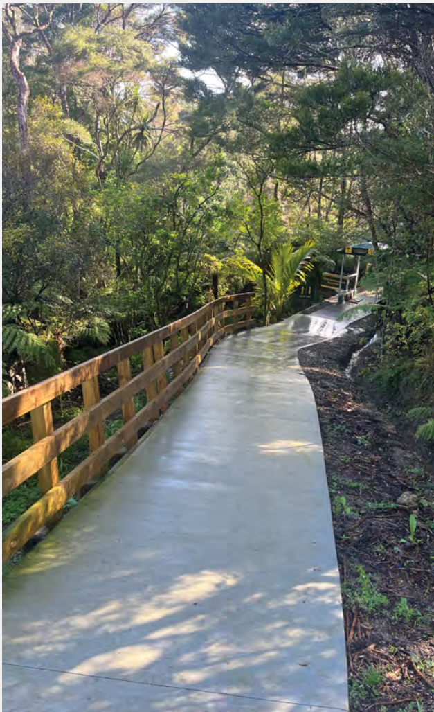
▲ Photo Steep path with concrete surface and handrail to enhance accessibility. Credit - Re Nature.
